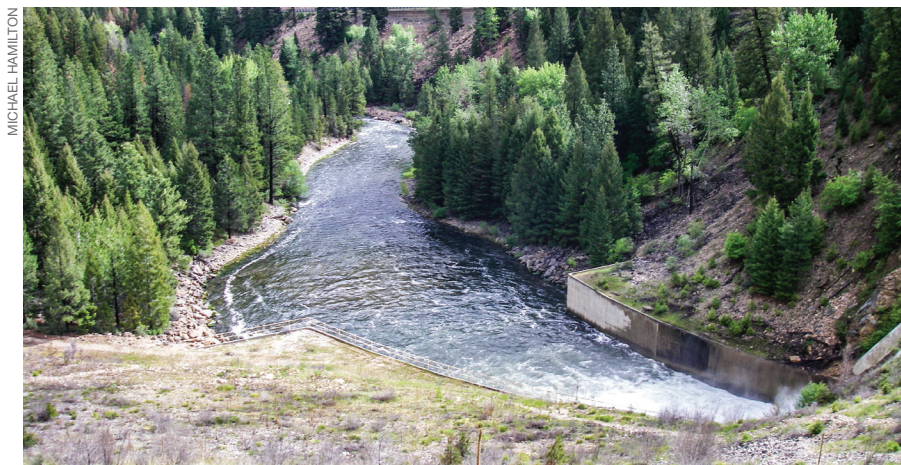
At full capacity, Painted Rocks Reservoir (top) can hold 45,000 acre feet of water, and because of the agreement in place, managers portion it out through a 143-foot high dam (bottom) throughout the year for both agricultural purposes and to add cool instream flows that help the Bitterroot's wild trout during years of low flows or high water temperatures.
